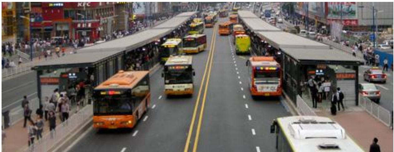
Figure 5 The Guangzhou bus rapid transit (BRT) system
